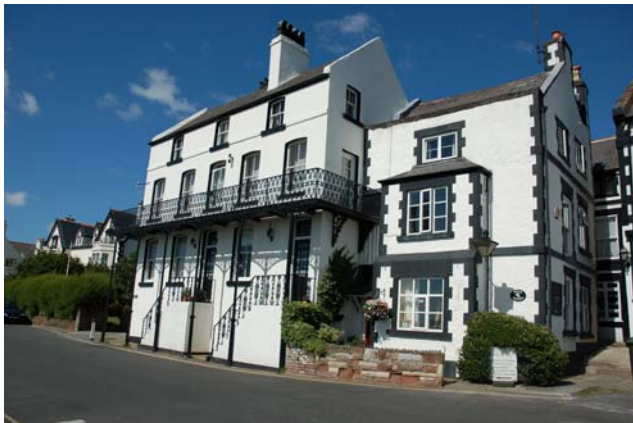
Balcony House, Parkgate
